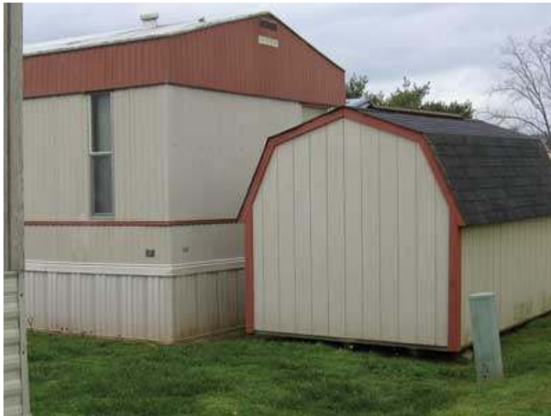
(15) This Dutch barn is covering most of a bedroom window. The window visible to the left may or may not open into the same room. If the first-in officer doesn't spot this hazard, the rapid intervention team should catch it and be sure to relay the information to the incident commander and interior crews.
