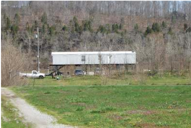
(7) This home, located in a flood plain next to a river, sits on concrete pillars approximately 10 feet tall. Note that there are no stairs outside the C-side door. You must include unusual hazards like this in your size-up and communicate them to all personnel.
