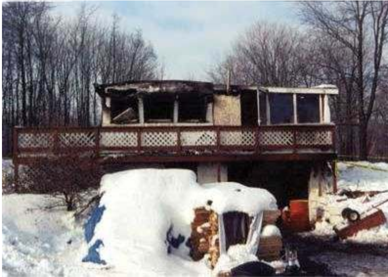
(4) This extensively modified manufactured home claimed the life of a 27-year-old lieutenant in Pennsylvania in 2001. This view of the B side shows the walkout basement and the end of a 43-foot-long enclosed porch, which was added to the A side. (Photo courtesy of the National Institute for Occupational Safety and Health, Line-of-Duty-Death Report F2001-04.)
