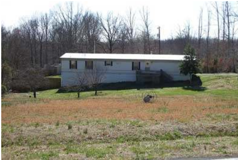
(6) Although the D side of this home is at ground level, the B side is essentially a second story.
